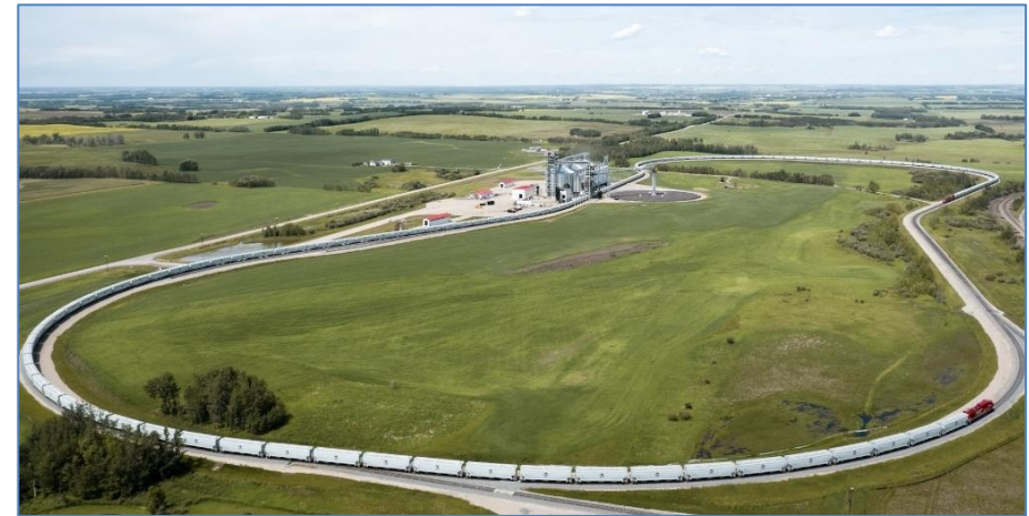
High-throughput elevators equipped with loop tracks, such as the Paterson Grain elevator situated at Bowden, Alberta, and shown here, have been instrumental in improving the efficiency with which grain moves through the GHTS in the past decade. Fifty-three such facilities can now be found across the Prairies. (Image courtesy of Paterson Global Foods)
