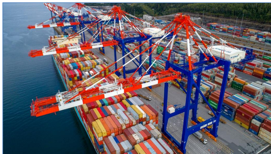
An aerial view of the Fairview Container Terminal located at Prince Rupert, British Columbia, and operated by DP World. The facility was purpose-built to serve the transpacific container trade, and features two marine berths capable of accommodating today's larger container ships. Designed for the direct ship-to-rail transfer of traffic, the adjacent intermodal yard is capable of handling trains up to 12,000 feet in length. (Image courtesy of Prince Rupert Port Authority)
