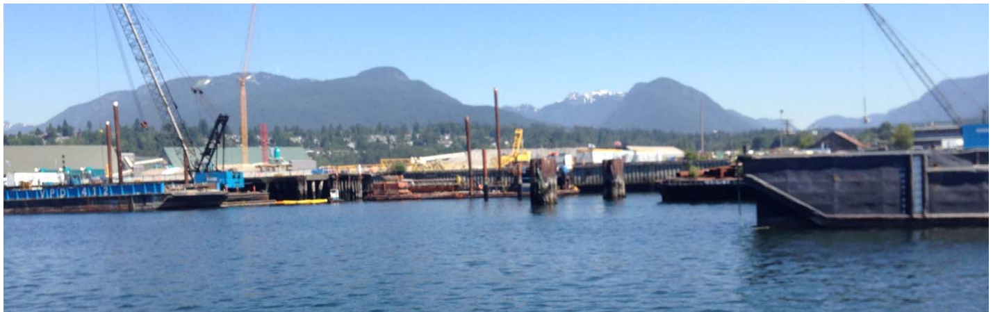
Construction of the G3 Terminal in North Vancouver (Quorum - July 2017)
