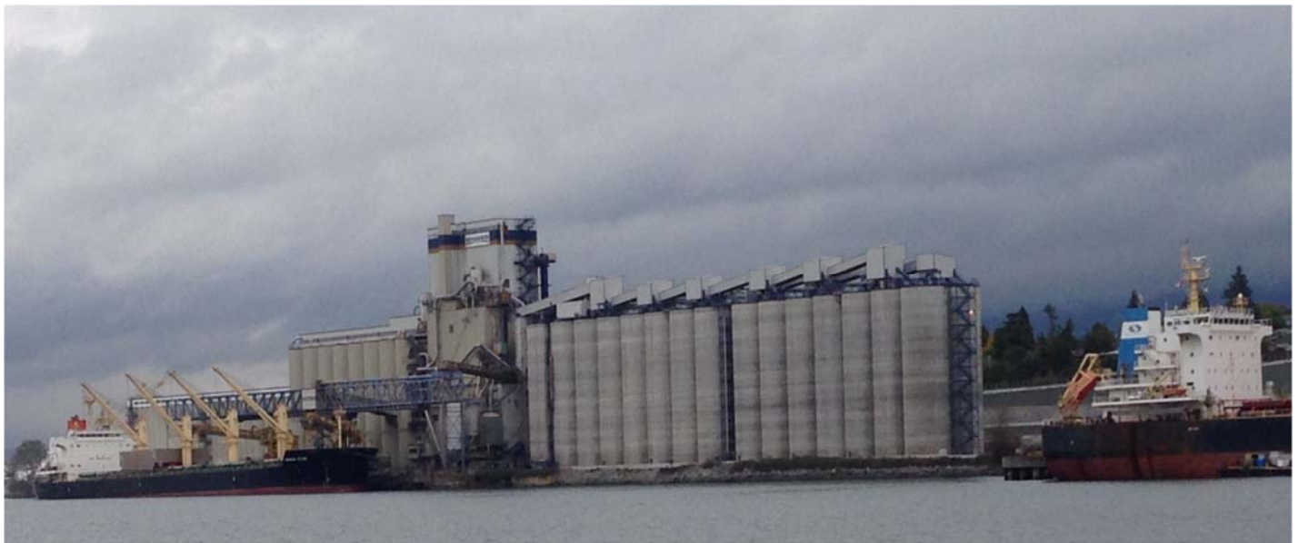
Richardson Terminal, Vancouver North Shore (Quorum, October 2016)
